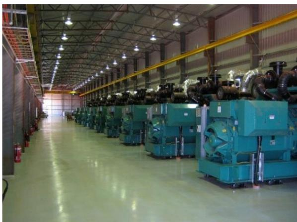
Figure 4 Typical Gas fuelled Engine Shed Layout
