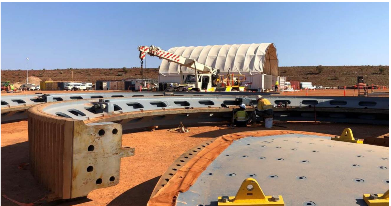
Figure 3: Assembly of the girth gear for the 36-foot diameter SAG Mill being assembled on site.
