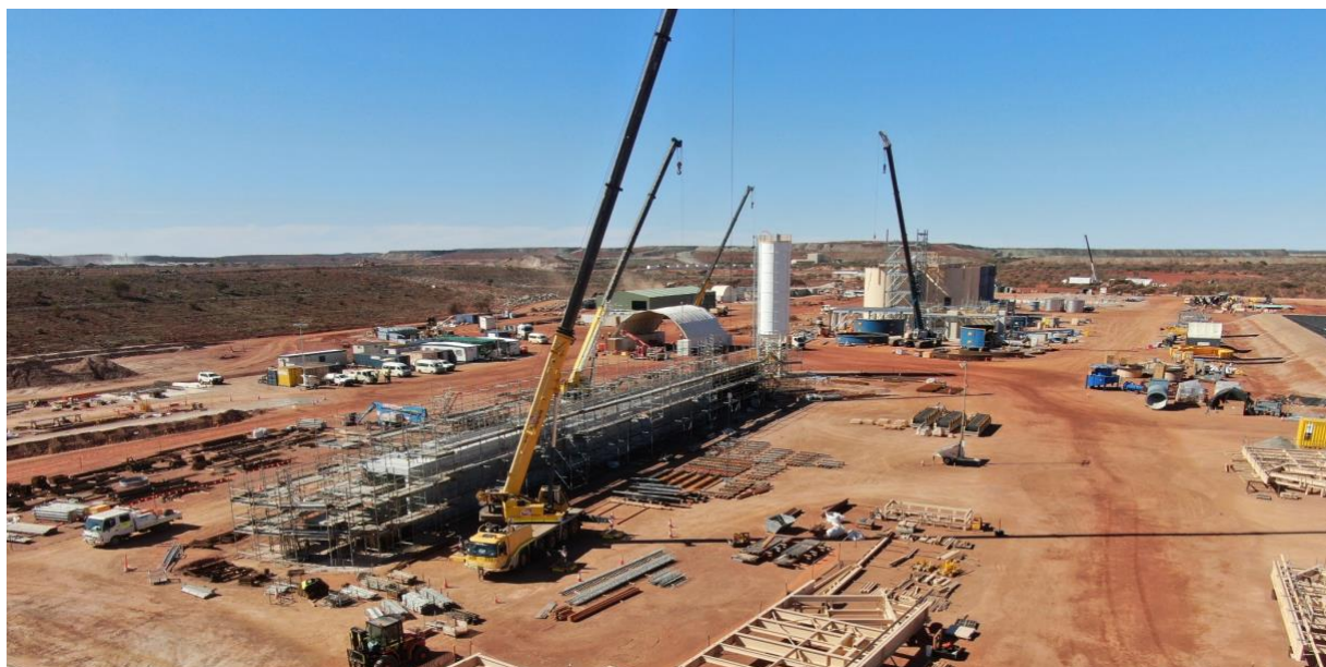
Figure 1: Stock reclaim tunnel (foreground) and process plant (rear) under construction.
