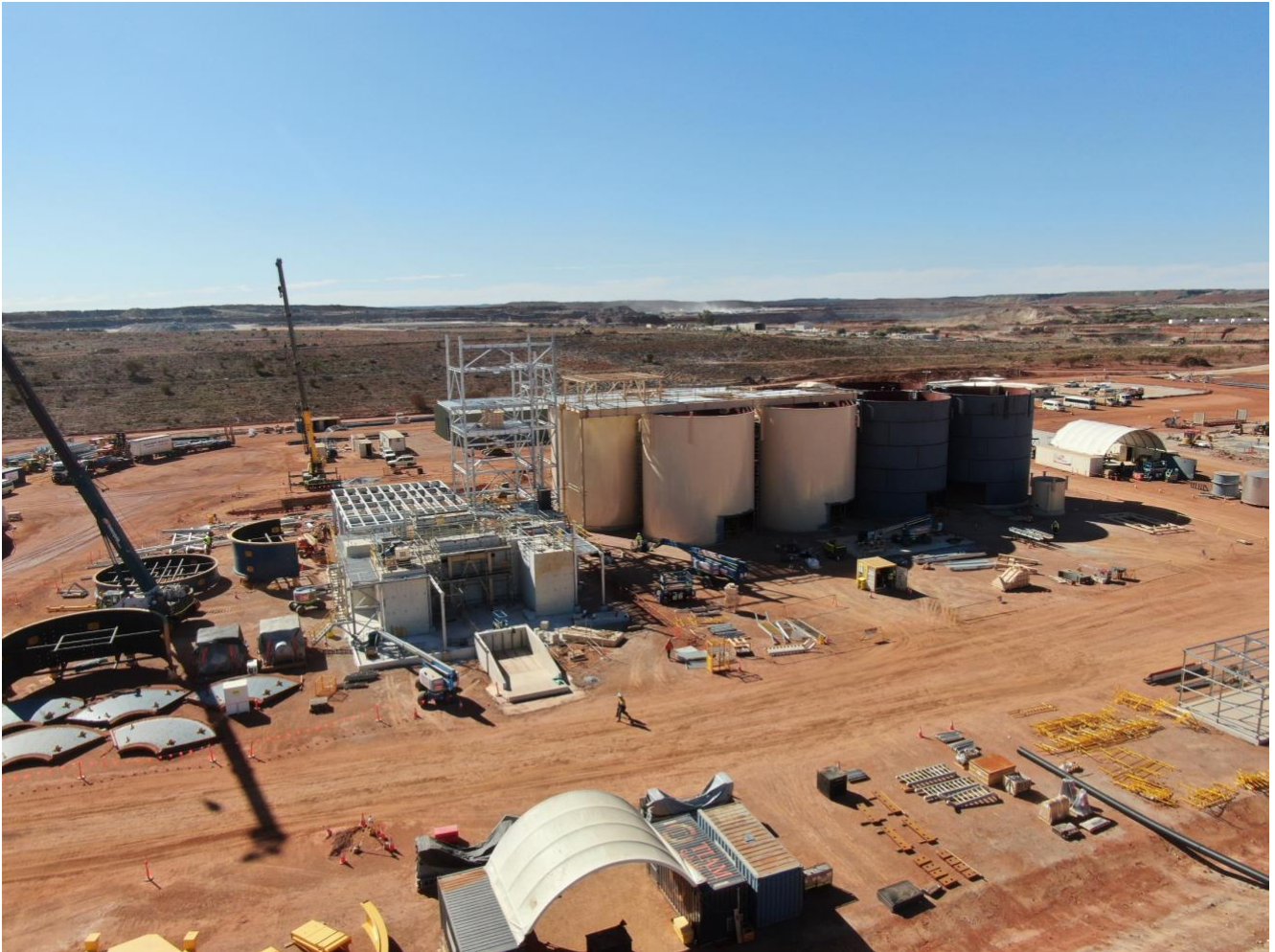
Figure 2: Processing plant and CIL tanks under construction.
