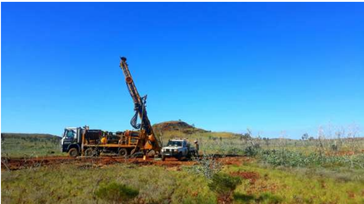
Figure 1: Reverse Circulation (RC) drill rig operating at the Fuego prospect, Croydon Project.
