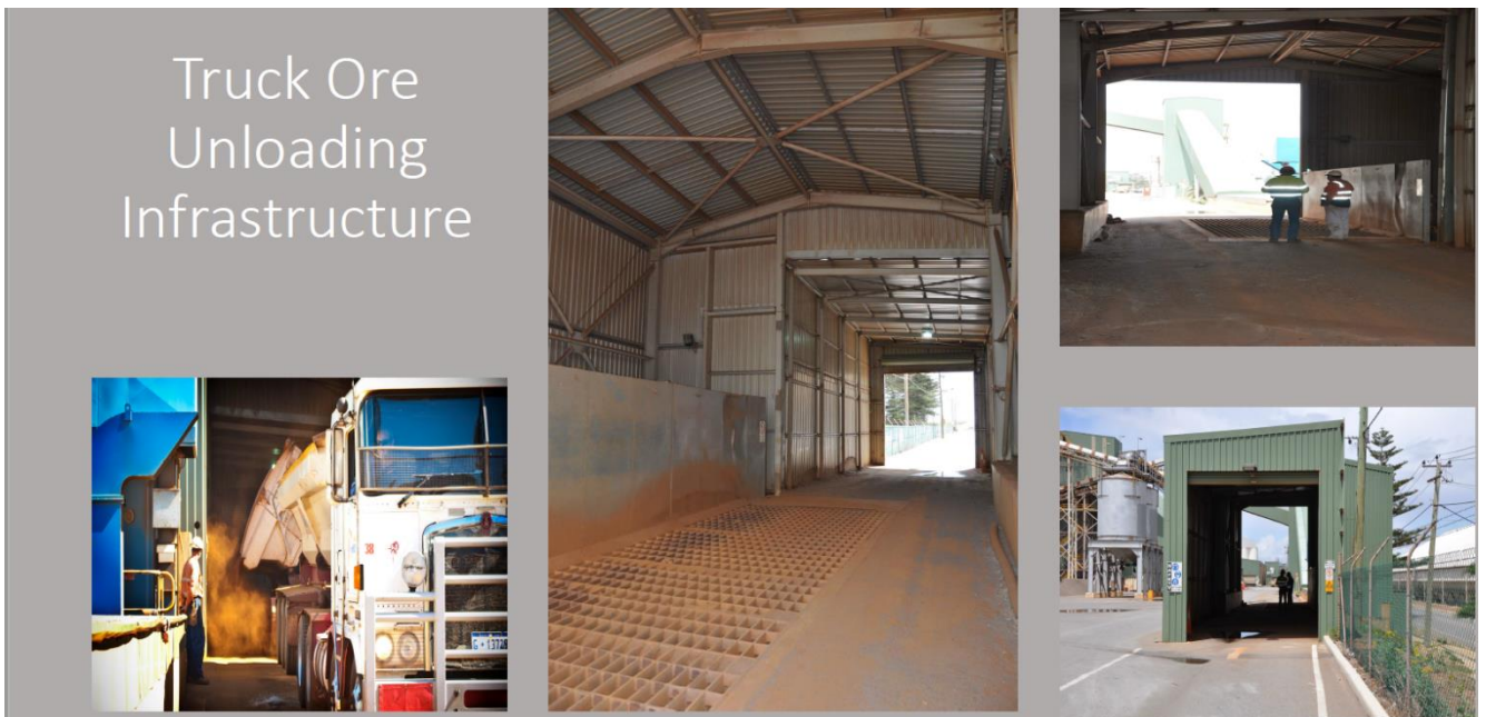
Existing Sinosteel Port Truck Unloading Infrastructure
