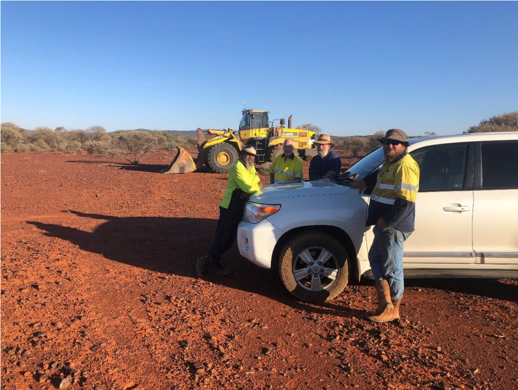
First pre-start meeting – Iron Ridge earthworks crew
