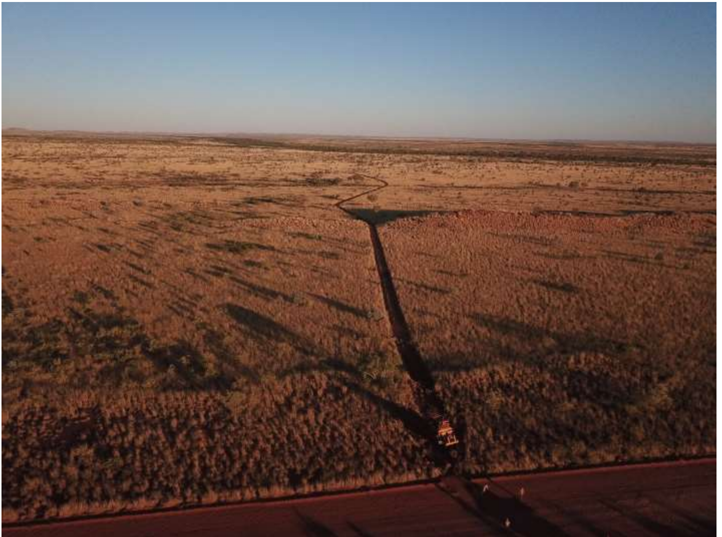
New access road construction commenced
